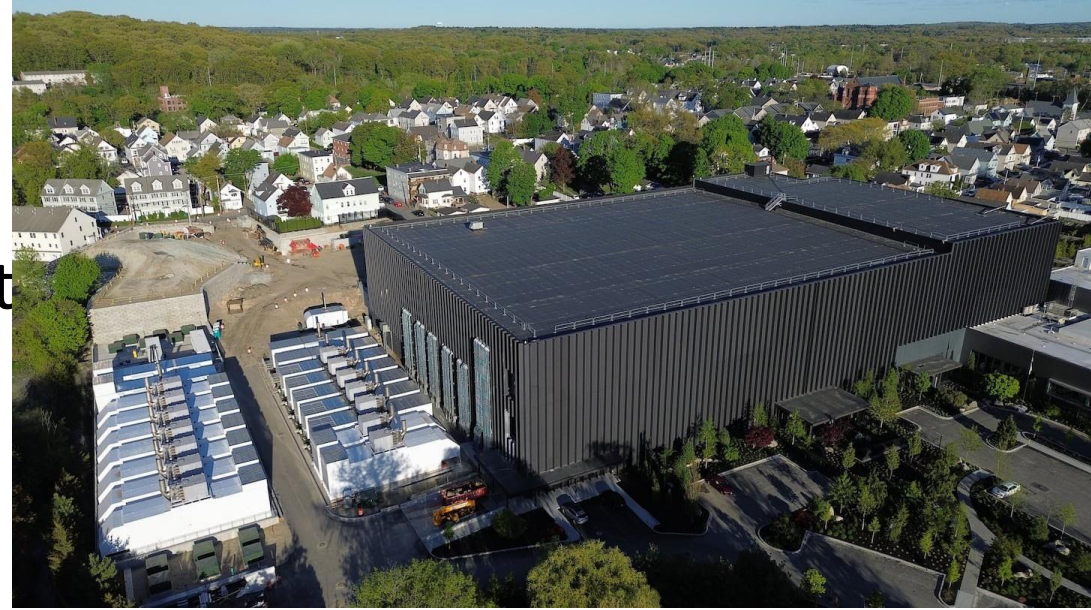
Above: Markley data center and diesel generators in Lowell, MA
